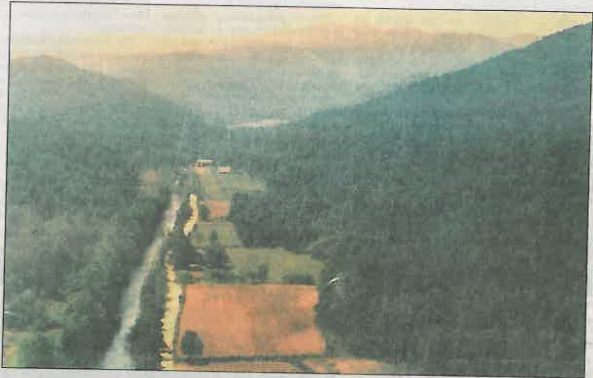
An aerial view shows Jocassee Valley, with the Attakulla Lodge visible at the end of the clearing.
